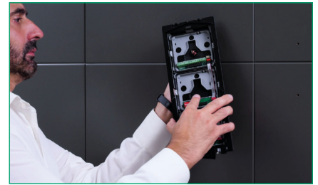
4. POSITION the surface-mounted entrance panel, guide the power supply wires through the appropriate slot and fasten it using the two screws at the top and bottom
