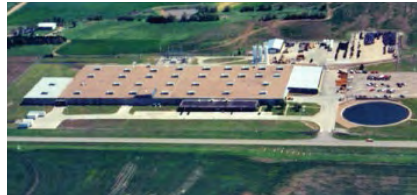
Hoisington Communications Plant | Hoisington, KS
