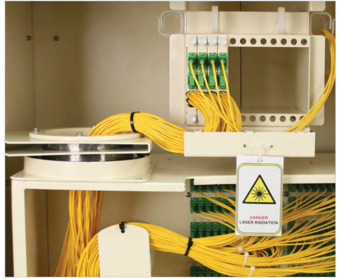
Fiber Management and Bend Radius Control
