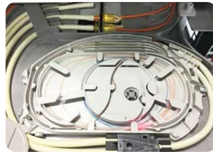
Macrobend easily visible in splice tray using 180XL
