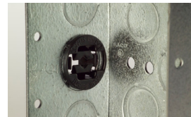
Step 2: Done - Ready for cable.
