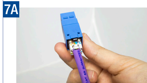
After cable is fully prepped, align your pairs in a 2 up, 2 down formation T568A: Green and brown pair up T568B: Orange and brown pair up
