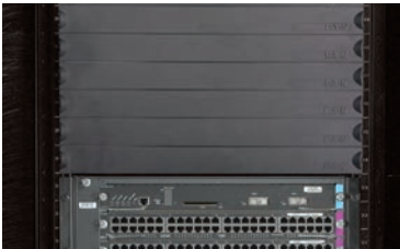
C Blanking panels are available to seal open U spaces.
