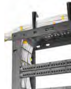
Wire Gates Installed
