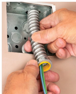
2 Screw connector into conduit. Snap assembly into box.
