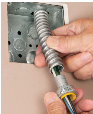
1 Pull flex conduit through 3/4" knockout in installed box.
