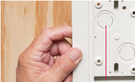
1 Disconnect electrical power. Remove knockout and insert supplied cable connector. Pull NM cable through connector.
