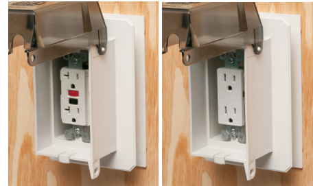
3 Install device, then the cover plate. The F8091 series works with GFCIs and most other single-gang devices. After siding is installed, caulk as required.
