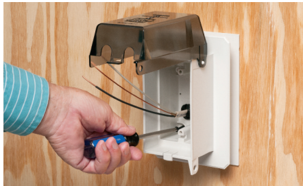
2 Attach box to substrate with screws.
