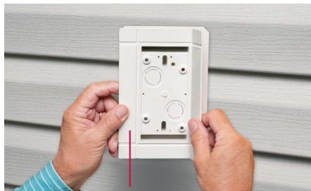
2 Break the flanges off of the back of the box. Remove knockout. Insert supplied connector and pull cable.
