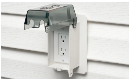
4 Install the single-gang device, then the cover plate.
