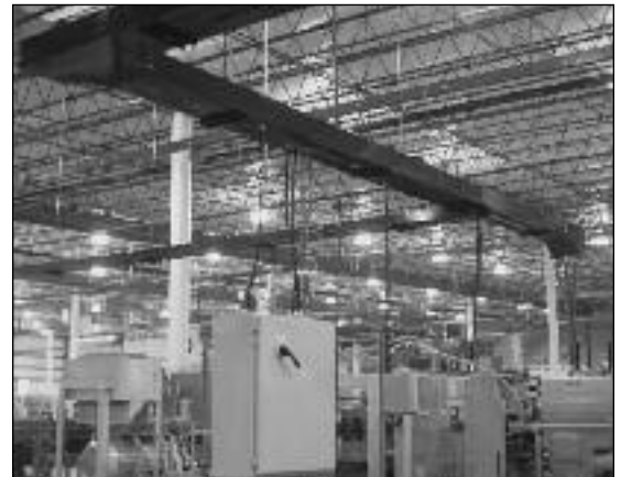
An overhead SpecMate Wireway installation in an industrial space.
