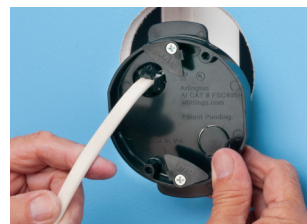
...Inserting it into installed NM94 connector. Tilt box to insert it into the stud cavity.
