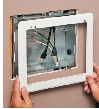
Attach plastic, paintable trim plate with screws provided.
