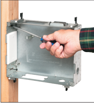
Mount box to stud, using tabs for proper positioning.
