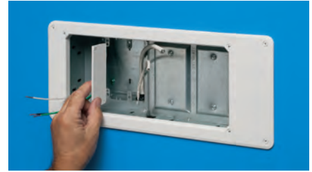
4 Install voltage separator.
