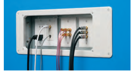
5 Install devices and plates.
