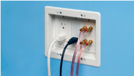
4 Install devices, then the wall plates.
