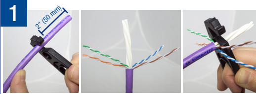
After cut, cross-web protrudes max. 0.04 in (1mm)
