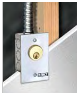
construction ready for easy wall installation
