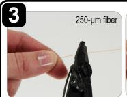
Strip 35 mm of 250-µm coating from the fiber.
