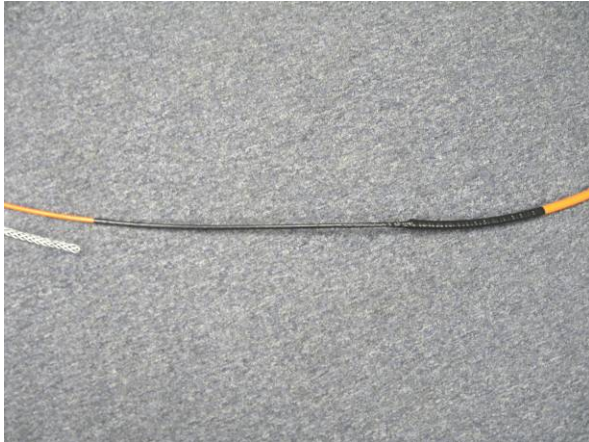
Figure 6: Apply tape from mark on inner cable to measured distance of the grip. At least 25% of the distance should cover the ILA or CST
