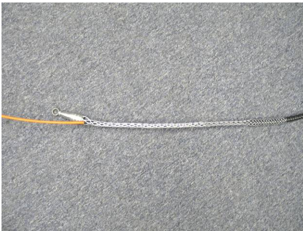
Figure 7: Pulling grip is inserted onto the cable assembly
