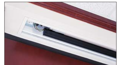
Bottom panel off during installation
