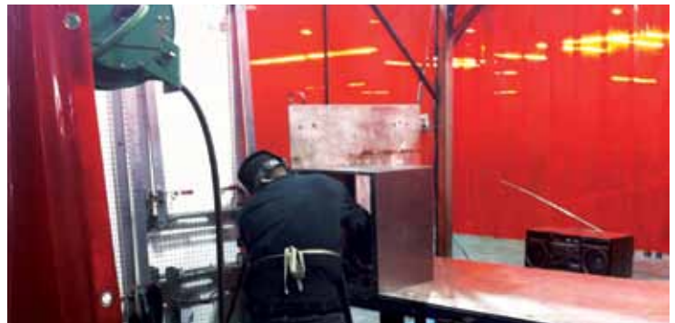
Welding Assembly in our Ennis, TX Facility
