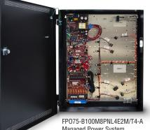
Managed Power System E2M enclosure, A-Wired Tie Wrap
