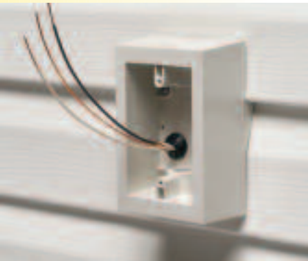
1 Pull wire. Attach the appropriate adapter to the FS8161T box and install on siding.
