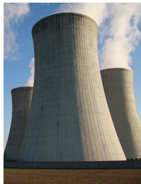
Figure 1. Cooling towers at a nuclear power plant
