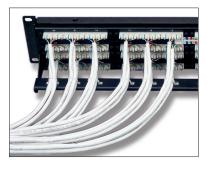
Integrated rear cable manager properly guides cables to and from the rear of the panel
