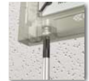
Concealed fixing screws already in position
