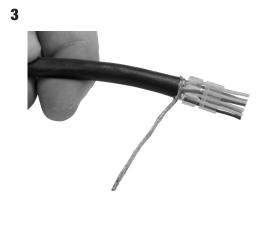
Separate all 4 pairs down to the pair spacer bar, align side by side making sure color code is correct. Insert conductors into load bar/liner.
