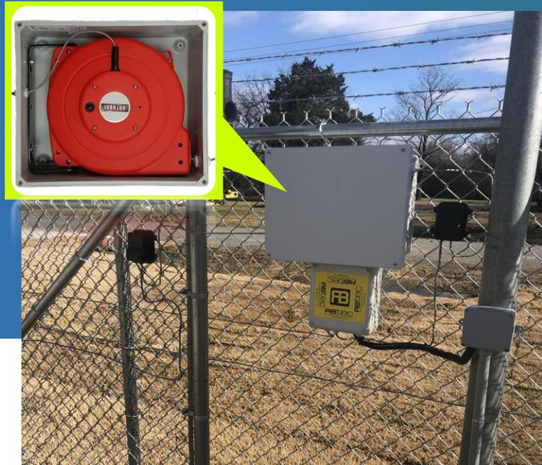
**Swing gate** – For swing gates there is no need for special equipment since the sensor cable is flexible. From the fence continue over the gate and do a U turn back to the fence. In order to bypass the gate the cable needs to be spliced with RG6 into a conduit and then spliced back on the other side. Splicing with RB-RBMCTXT Box
