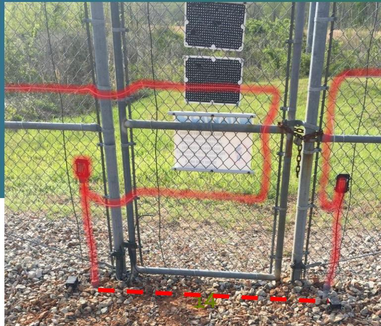
**Emergency gate / No Conduit** – For swing gates where there is no conduit or the gate rarely opens there is an option to splice the cable and install a pull out quick connector which allows to open the cable and as a result open the gate the cable is going over.
