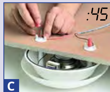
C Two (2) standard wire nuts connect the speaker wires to the mounting studs, making the electrical connection. That's all it takes!
