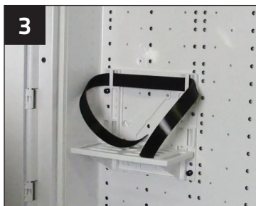
3 Optional mounting tape to secure hardware. (not included)
