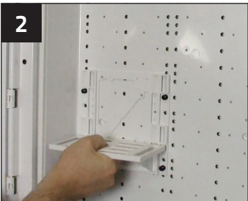
2 Mount shelf into place and secure.
