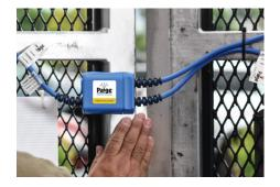
Reconnect male and female Perimaguard Asset Protection Loop components and test mount so as to determine where to thread the wiring.
