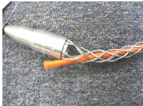
Figure 10: Excess Cable Pulled Through the End of the Pulling Grip
