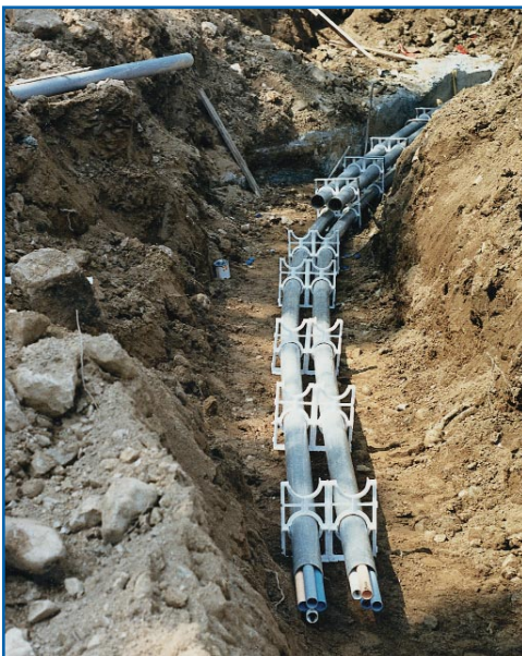
Pulled through existing conduits
