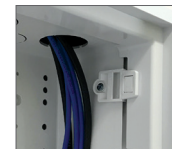
Installed SMC for affixing sidewall to stud.
