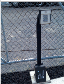
At the base of a pole
