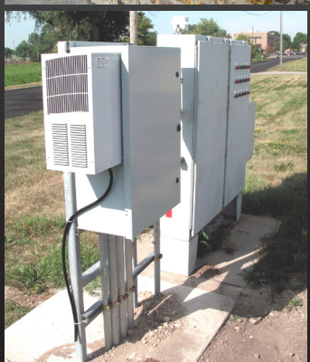
Using metal tubing or angle-iron and a concrete slab
