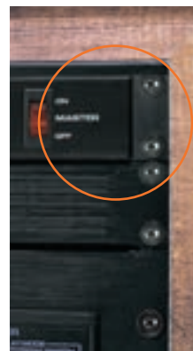
without trim strip installed
