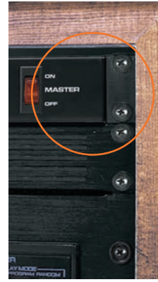
without trim strip installed
