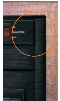
without trim strip installed
