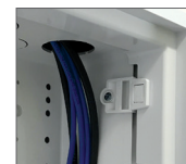
Installed SMC for affixing sidewall to stud.
